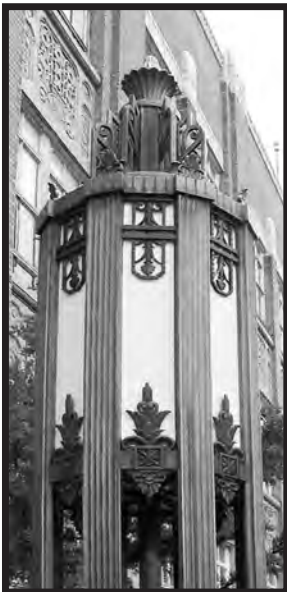
Light fixture decoration
